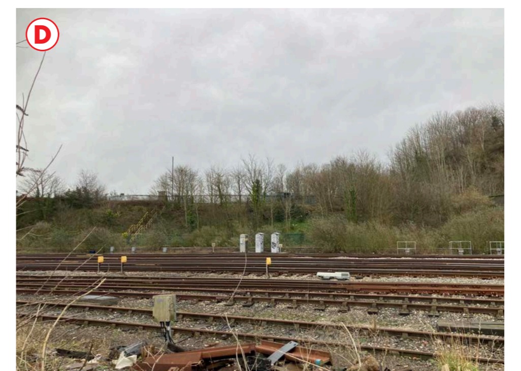
View towards site looking south across mainline railway
