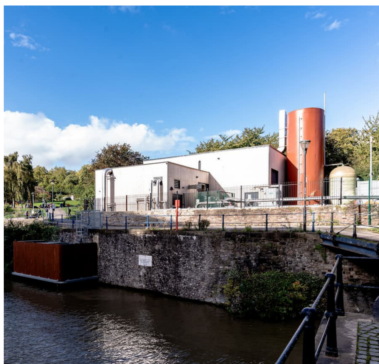
Castle Park Energy Centre, another Vattenfall scheme that already supplies the network
