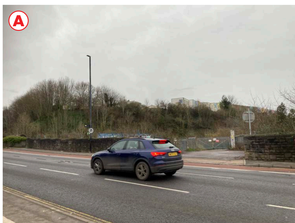
View into site entrance from across Bath Road
